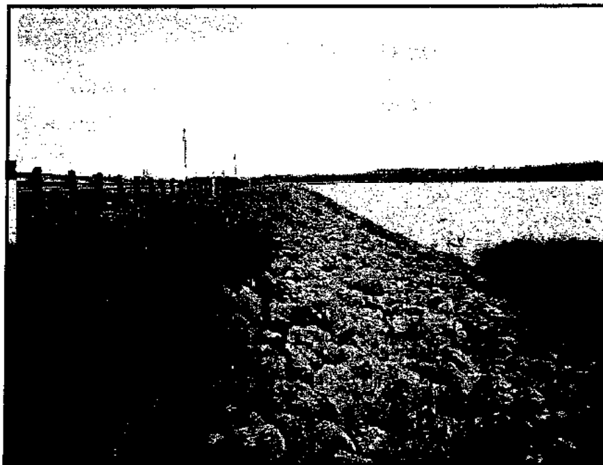
Photo 2: Upstream embankment and rip-rap
